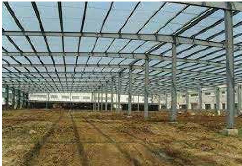
Bondada Industrial Park, Rampally
